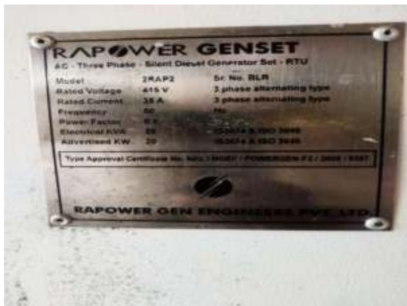
(a) Generator Installed
